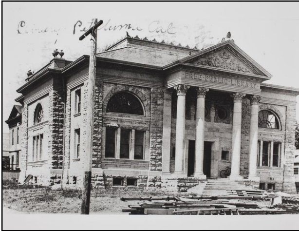
Petaluma Carnegie Library under construction circa 1905
