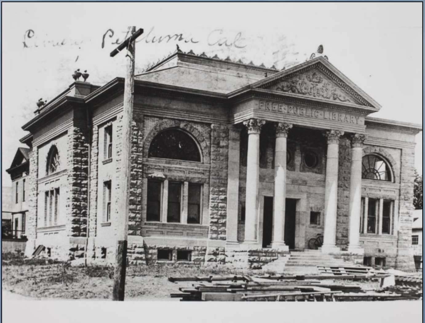
Petaluma Carnegie Library under construction circa 1905
