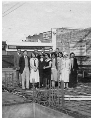
Sonoma County National Bank under Construction, 1925
