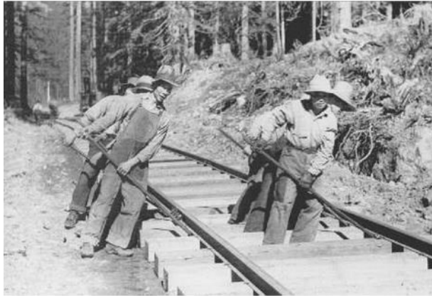
Chinese labor laying tracks
